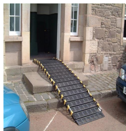
Roll-a-ramp at the Millworkers House
