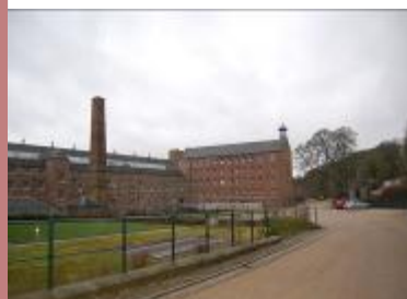
Mill Square and the Mid Mill and Bell Mill, Stanley Mills.
